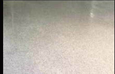
With Fiber No Crack
